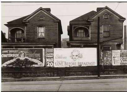
Houses and Billboards in Atlanta 1936 © Walker Evans
